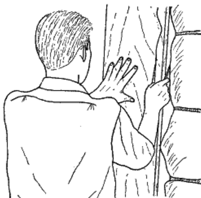
FIG. 95.—Marking a board to fit against an irregular rock wall. By means of the dividers, a mark is made on the board parallel to the surface of the wall.
